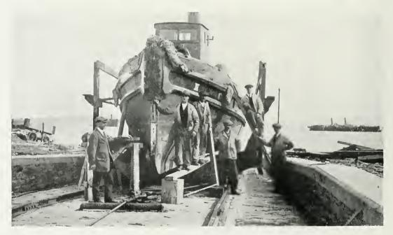
REPAIRING A STEAM PINNACE ON THE SLIPWAY AT LYNESS.
